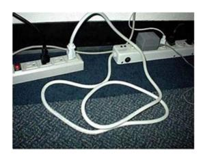
Relocatable power taps shall be directly connected to a permanently installed receptacle.  Relocatable power taps shall be of the polarized or grounded type, equipped with overcurrent protection, and shall be listed in accordance with UL 1363.
